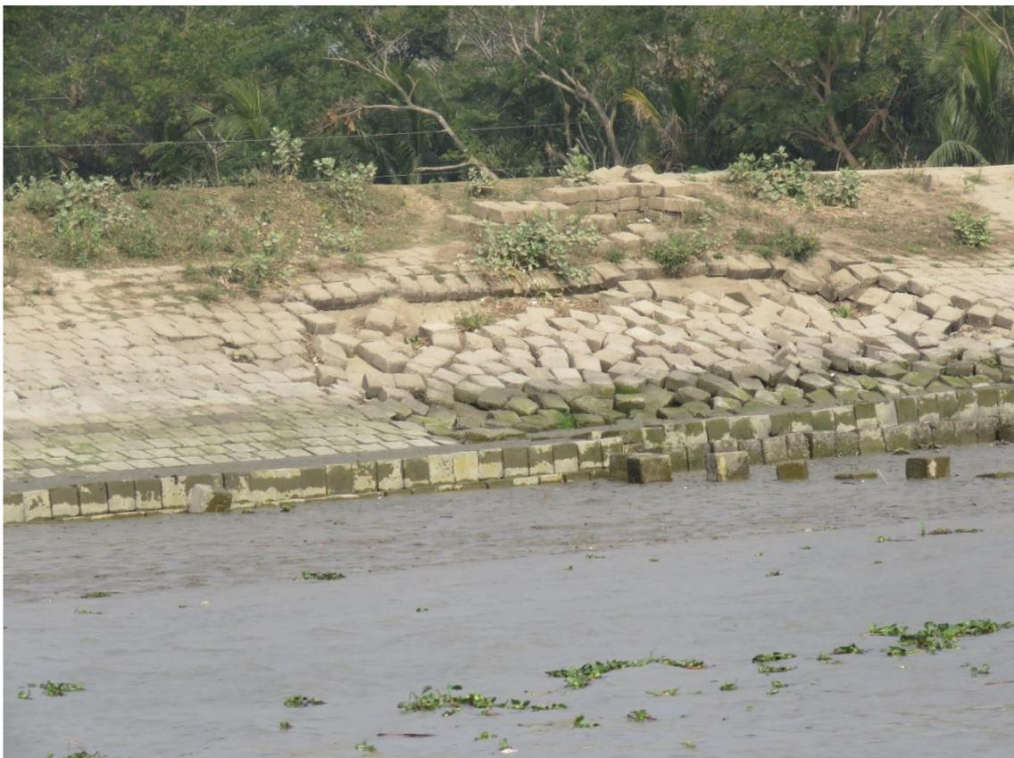
Figure 4-5: Bank erosion along the Baleswar river, photo from field conducted 10 February 2019.
