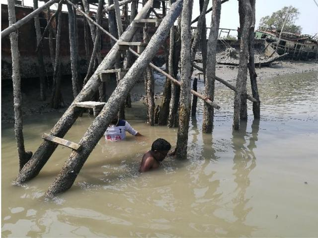
Figure 2-2: Installation Pressure sensor for water level recording during bathy survey at inside Sundarbans
