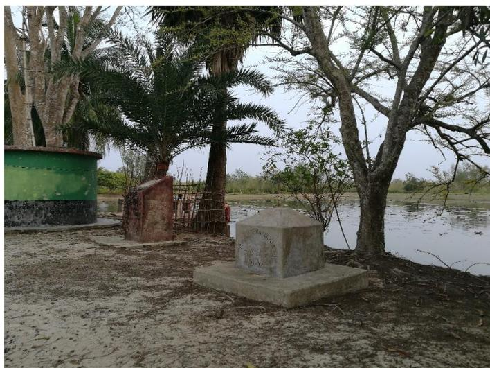
Figure 2-1: SOB Benchmark at Kapilmuni (Sundarbans) used for Bathymetry
