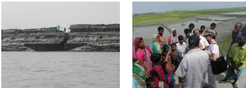
Photo-1: Settlements Built on the Sibsa embankment in Polder 32
