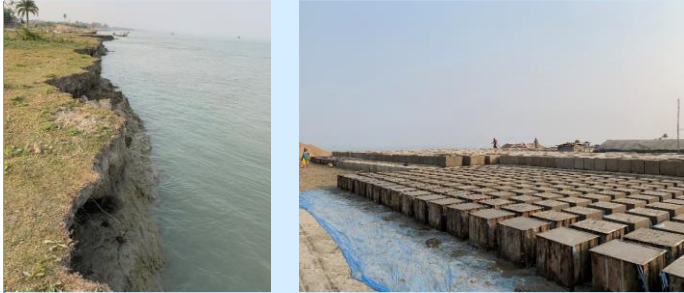
Photo 10: River erosion at the eastern shoreline at Char Fasson of Bhola Island. Photo 11: CC block for erosion mitigation.
