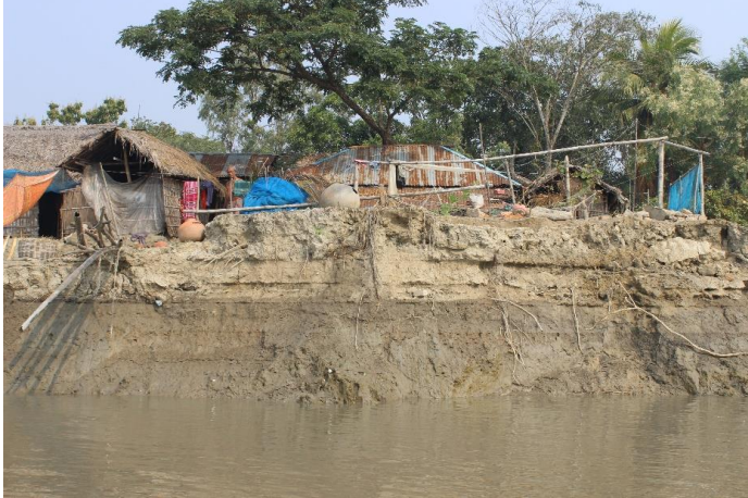
Photo-4: River Erosion of Polder 29, 2016
