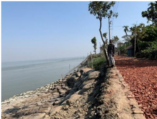
Photo-12: Strengthening of embankment to avoid overtopping during cyclone
