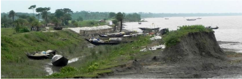
Photo-2: Damage by Cyclone Sidr on Polder 35/1 on Baleswar River
