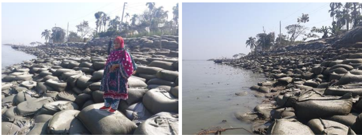
Photo-13: Sand-filled geo-bag at Daulatkhan
