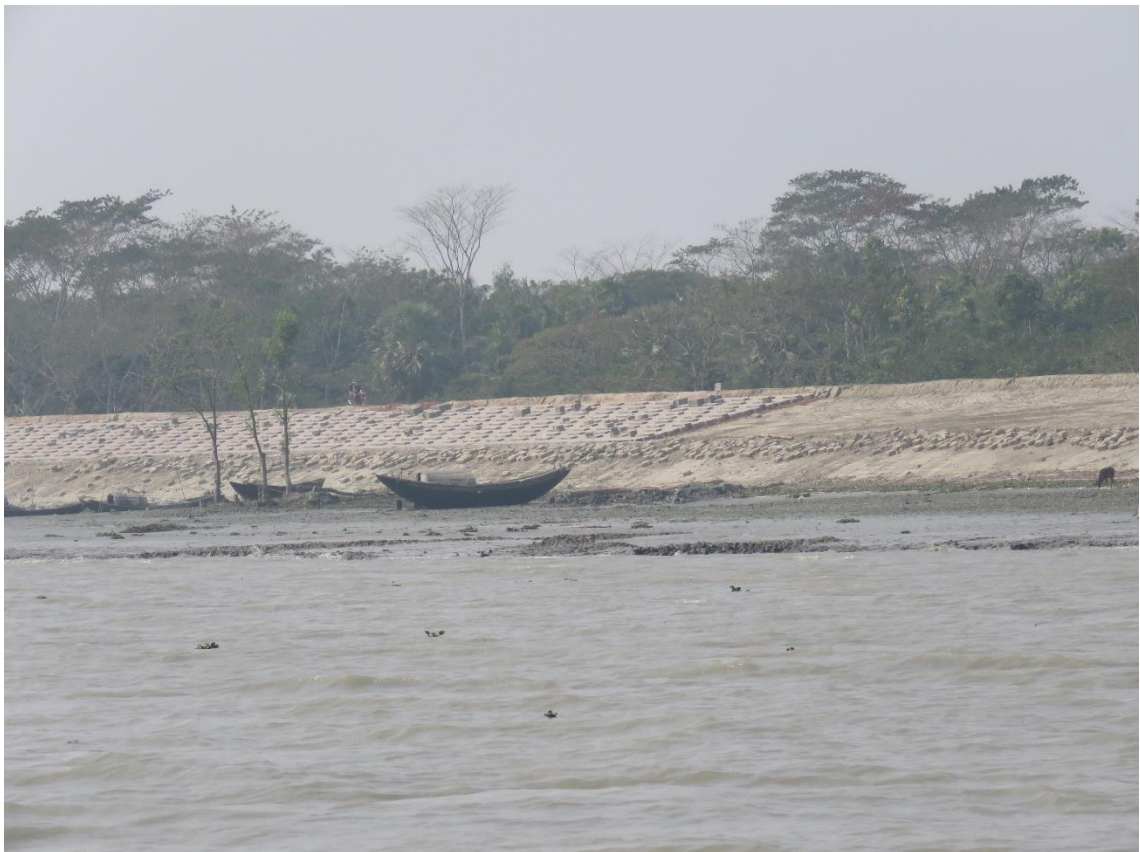
Figure 1-1 Revetment along Baleswar River (photo 11 February 2019).
