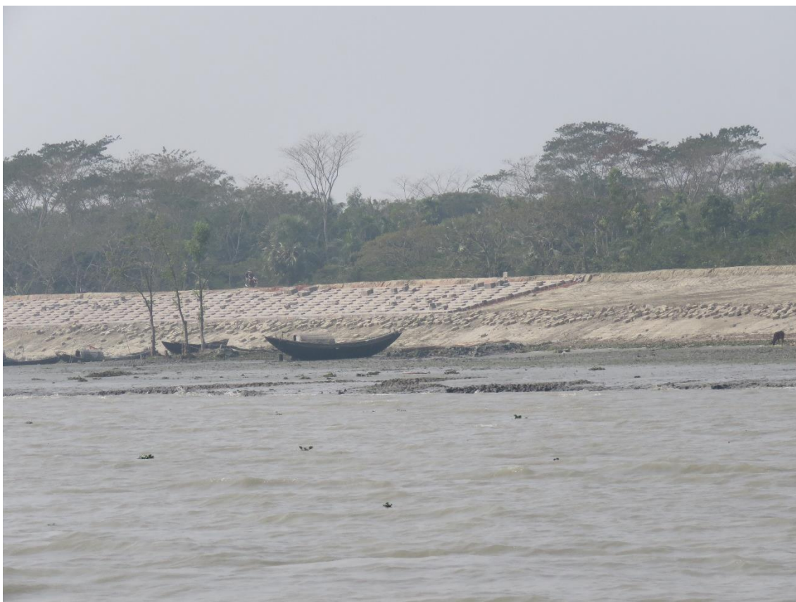
Figure 1-1 Revetment along Baleswar River (photo 11 February 2019).
