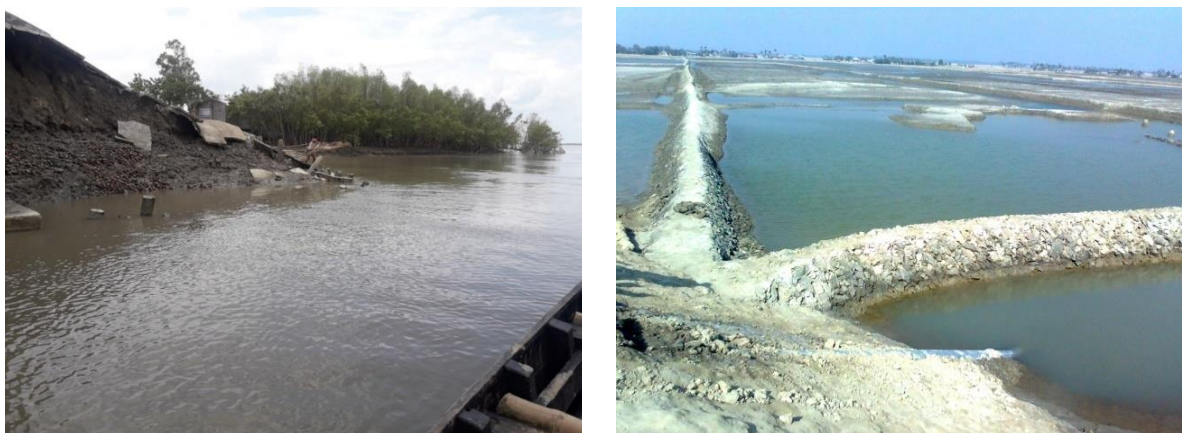
Figure 4: River bank erosion and Fish ghers in the Polder 14/1 and Polder 15
