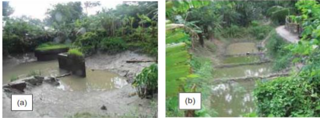
Figure 8: Present condition of existing regulators (a) Keukhali sluice and Cross dam in Sutanalir Khal (b)
