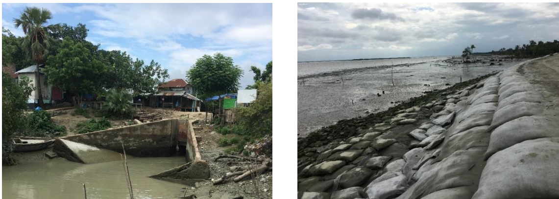
Figure 6: Repaired damaged regulator and erosion protective work in Polder 40/1
