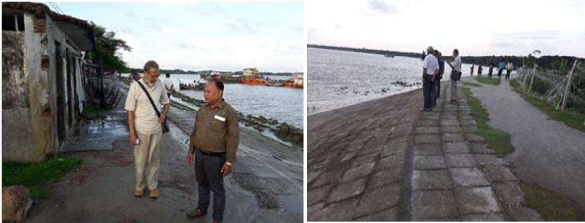
Figure 13: Bank protection at Kamalgonj area and upstream termination
