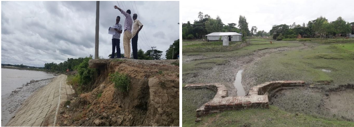
Figure 9: Eroded river bank with bank protection work and sedimented khal with broken structure in the Polder 64/1b
