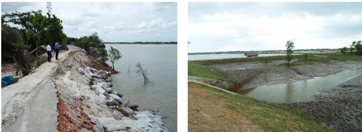
Figure 16: River bank erosion and siltation problem in the Polder 29
