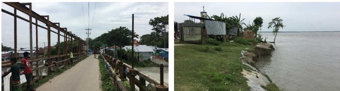
Figure 20: Existing sluice gate condition (Boalia) and erosion prone location at Panpatty Bazar in Polder 55/1.
