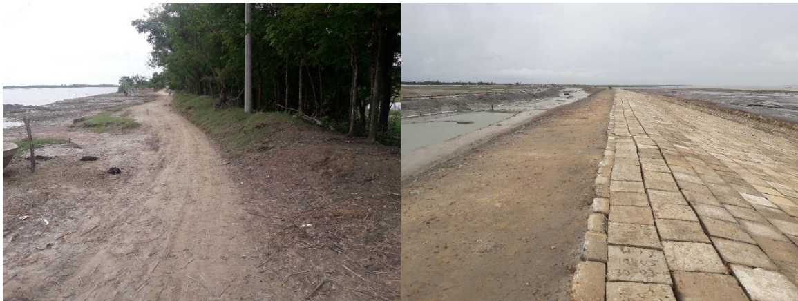
Figure 10: Broken embankment and sea-dyke protection work in the Polder 64/1a
