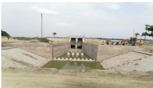
Ongoing DS-3 In Polder-43/2C
