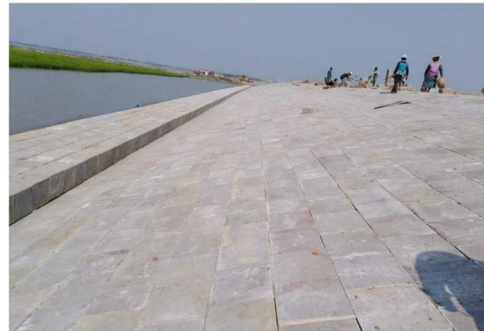
Completed Slope Protection Works in Polder-32
