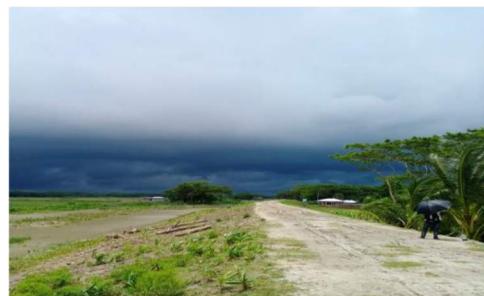
Embankment work from Km 9+800 to Km 11+000 in Polder-43/2C
