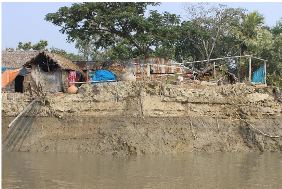
Photo-4: River Erosion of Polder 29, 2016
