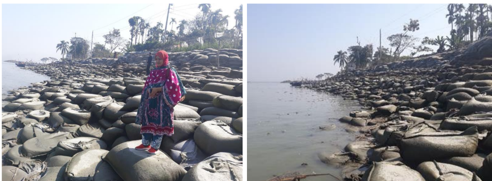
Photo-13: Sand-filled geo-bag at Daulatkhan
