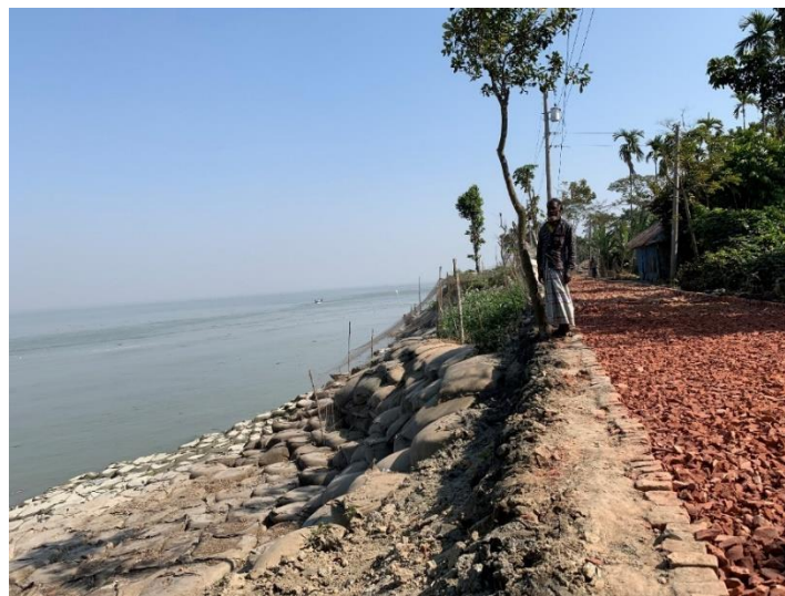
Photo-12: Strengthening of embankment to avoid overtopping during cyclone
