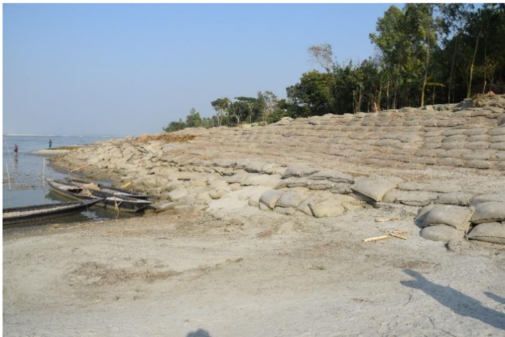
Photo-7: River bank protection by sand fill Geo-bags
