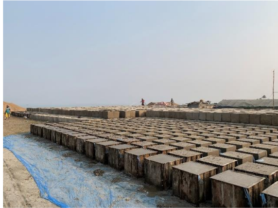
Photo 10: River erosion at the eastern shoreline at Char Fasson of Bhola Island. Photo 11: CC block for erosion mitigation.
