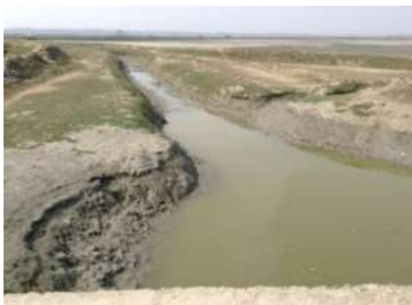
Photograph 6.5: Deteriorated drainage khal in D/S-2 and D/S-1
