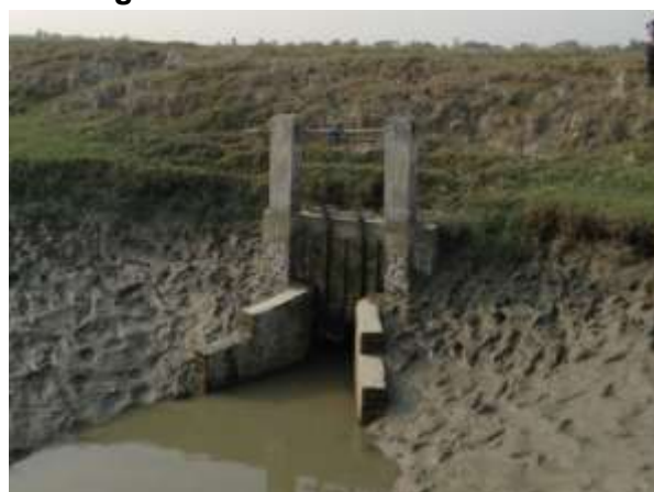
Photograph 5.6: Deteriorated condition of F/S-29
