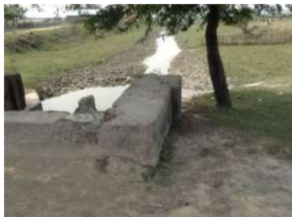
Photograph 6.5: Deteriorated drainage khal in D/S-2 and D/S-1
