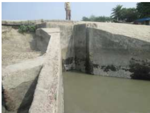
Photo 5.3: Deteriorated condition of DS-2
