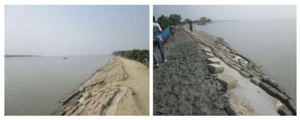
Photograph 5.2: Deteriorated Condition of Existing Slope Protection Work
