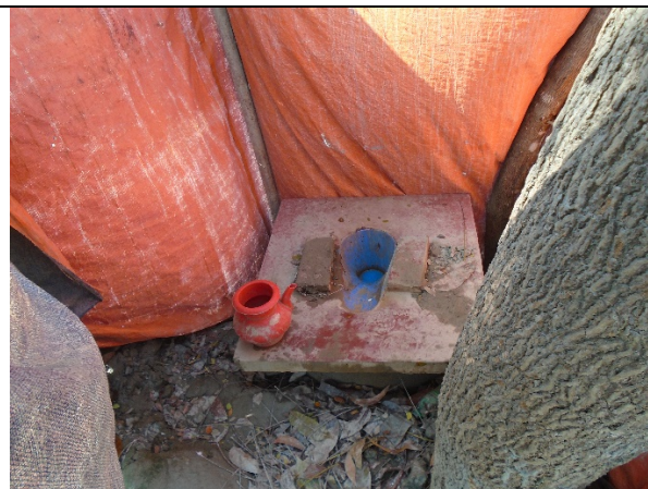
Latrine without water seal in DS-06, under polder no. 43/2C
