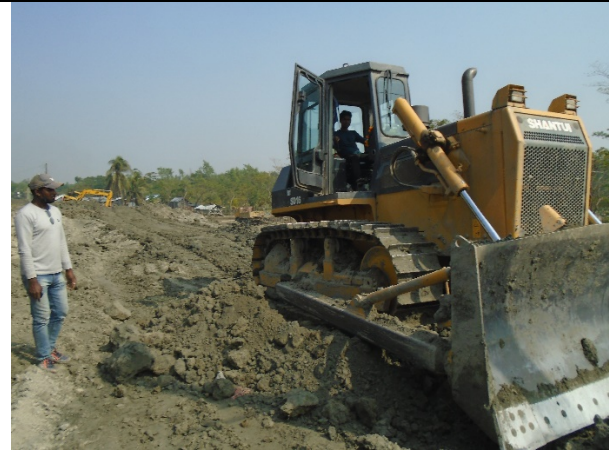
Without any ear plug the driver operates the high noise vehicle under polder no. 40/2
