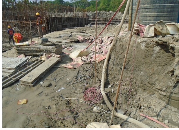
Electric wire on the ground in worksite of DS-06, under Polder no. 43/2C
