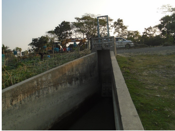
Flushing Sluice (FS)- in the polder no. 41/1
