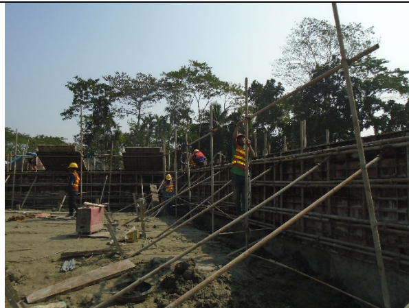
Without using PPE worker work in the of DS-6, under Polder no. 43/2C
