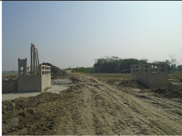
Drainage Sluice (DS)-02 Structure work has been completed but not yet operational, polder no. 43/2C
