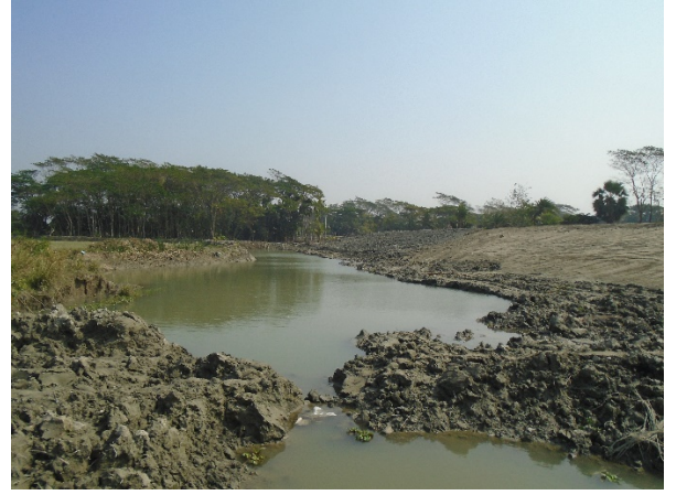
Not maintain the minimum distance from borrow to toe in chainage km24.800 under polder no. 43/2C
