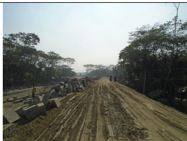
Without proper signboard and any demarcation Slope Protection Work (Ch: km 23.512) is ongoing under polder no.-35/1
