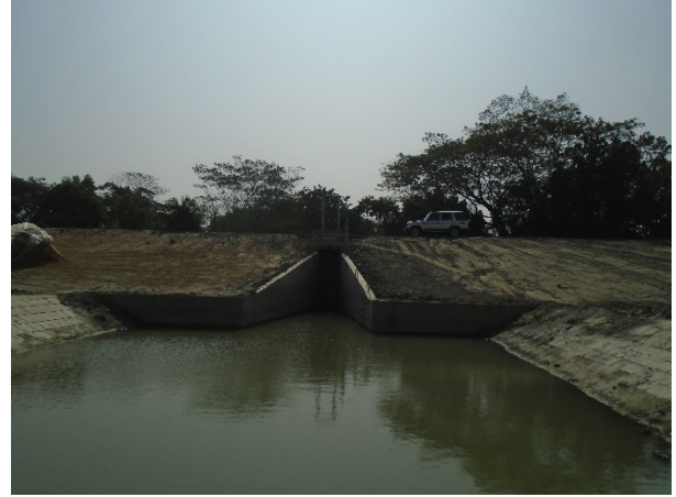
Flushing Sluice (FS)-1A in polder no. 43/2C
