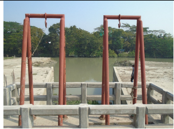
Drainage Sluice in the polder no. 40/2
