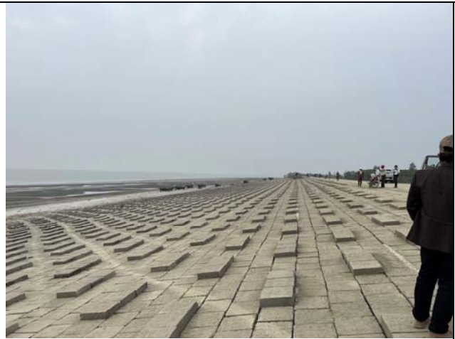
View of completed slope protection works at Kuakata of polder 48
