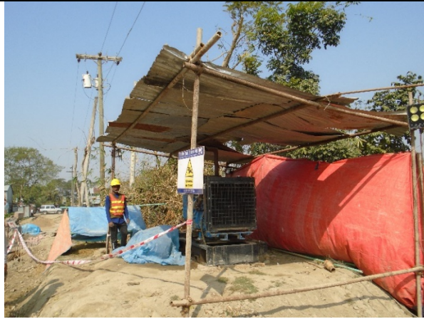
Generator with no secondary containment at DS-06, under Polder no. 43/2C
