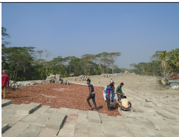
Workers without using PPE at Slope Protection Work (Ch: Km 23.512) under polder no.-35/1
