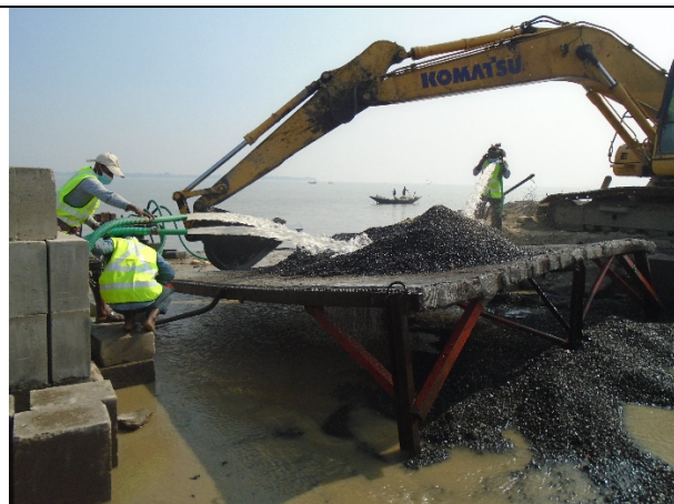
Stone washing o the river bank at Tafal bari CC block manufacturing yard under polder no.-35/1
