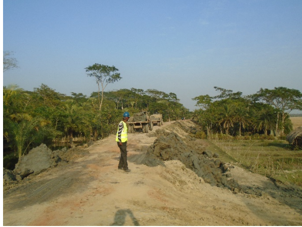
Without proper signboard and any demarcation Embankment Work (Ch: km 52.250) is ongoing under polder no.-35/1
