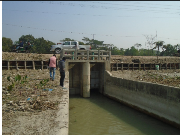
Drainage Sluice (DS)-9 in the polder no. 40/2
