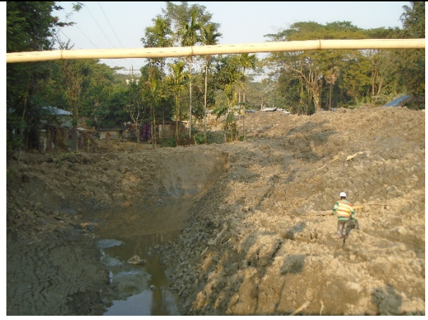
Collecting soil for construction of embankment (chainage: 27.000) and deep excavation in the locality side under polder no. 41/1
