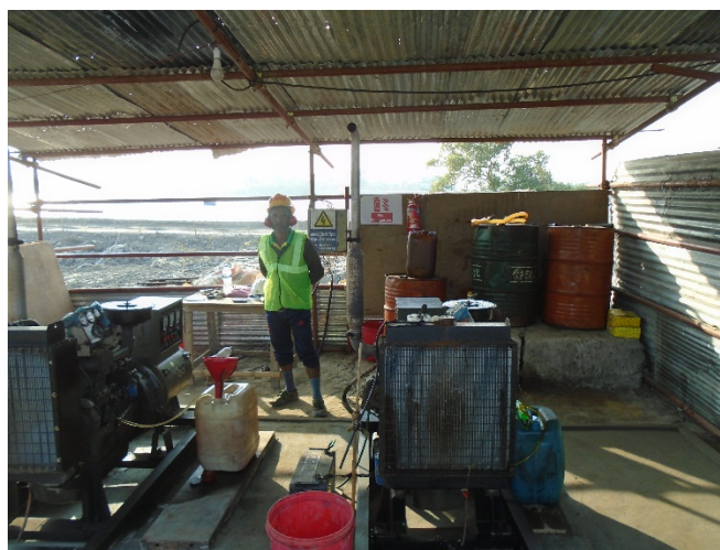
Generator on paved floor with bundh
