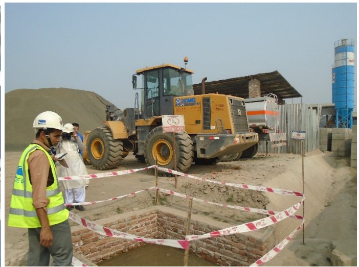
Waste water Decanting ponds in CC block manufacturing yard
