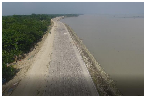
Figure 3-10: Completed Slope Protection Works in Polder-32
