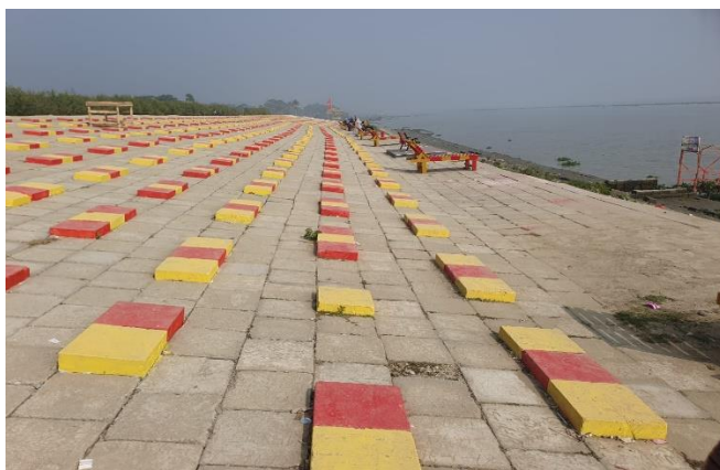
Figure 3-11: Completed Slope Protection Works in Polder-35/1
