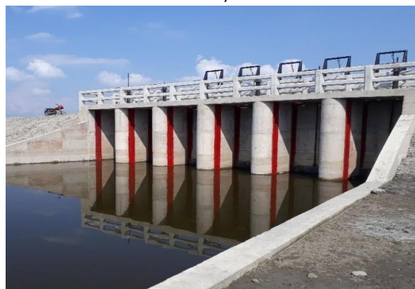
Figure 3-13: Completed 6 vent DS of Polder-35/3
