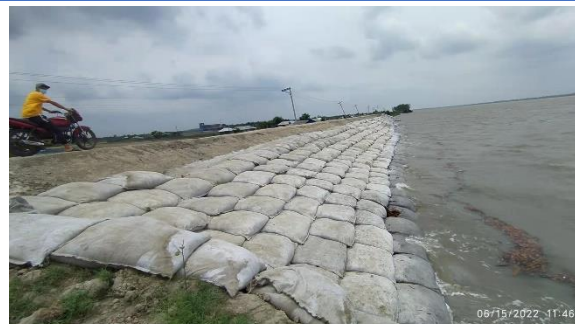
Figure 3-14: Emergency Works of Polder-32
