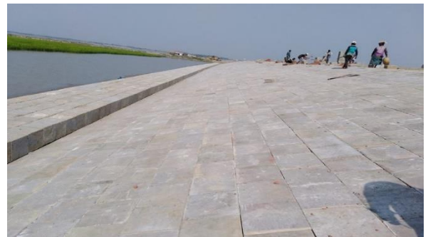
Figure 3-10: Completed Slope Protection Works in Polder-32
