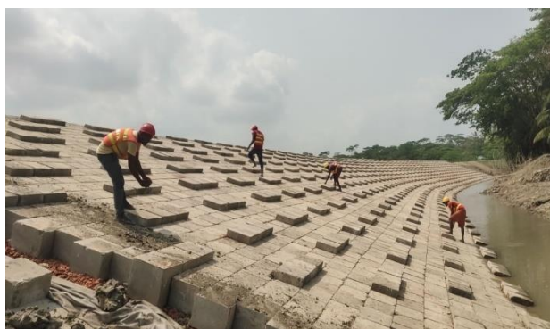
Figure 3-25: Slope protection work for km 32+015-34+300 in Polder-39/2C
