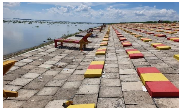
Figure 3-12: Completed Slope Protection Works in Polder-35/1
