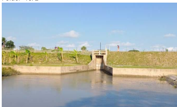
Figure 3-26: Complete Drainage Sluice DS-1 in Polder-40/2
