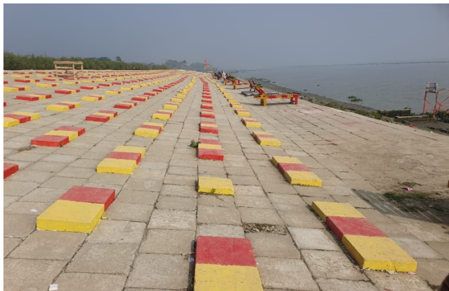
Figure 3-11: Completed Slope Protection Works in Polder-35/1
