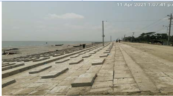
Figure 3-28: Slope Protection work from KM 30+800 to Km 31+450 in Polder-48
