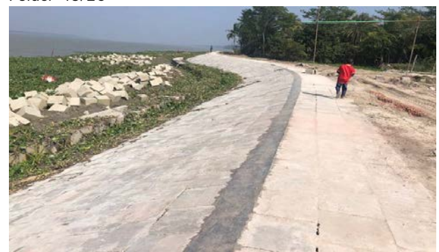
Figure 3-27: Slope & Bank Protection work in Polder-39/2C
