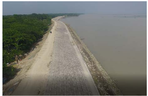
Figure 3-10: Completed Slope Protection Works in Polder-32
