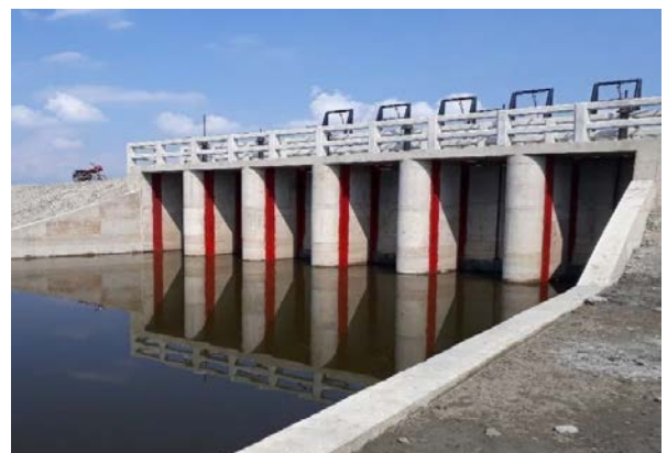
Figure 3-13: Completed 6 vent DS of Polder-35/3
