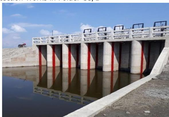
Figure 3-13: Completed 6 vent DS of Polder-35/3
