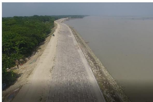
Figure 3-10: Completed Slope Protection Works in Polder-32
