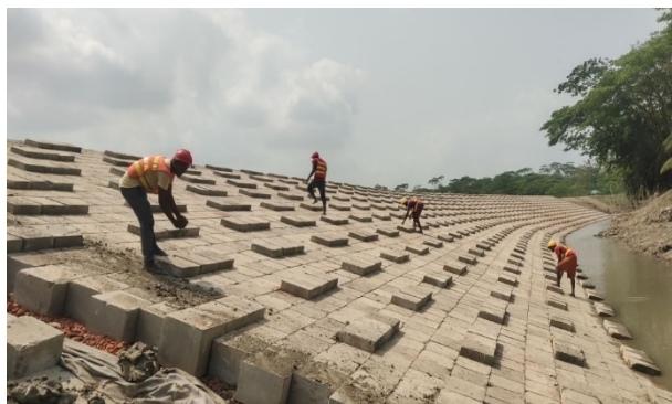
Figure 3-25: Slope protection work for km 32+015-34+300 in Polder-39/2C
