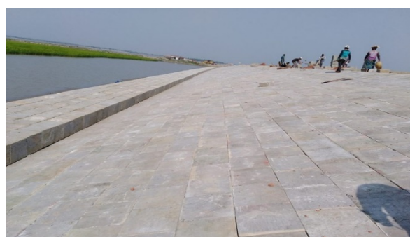
Figure 3-10: Completed Slope Protection Works in Polder-32
