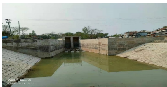
Figure 3-25: Slope protection work for km 32+015-34+300 in Polder-39/2C
