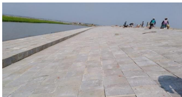
Figure 3-10: Completed Slope Protection Works in Polder-32
