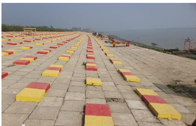
Figure 3-11: Completed Slope Protection Works in Polder-35/1
