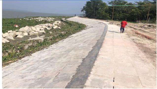
Figure 3-33: Slope & Bank Protection work in Polder-39/2C
