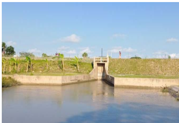
Figure 3-27: Complete Drainage Sluice DS-1 in Polder-40/2
