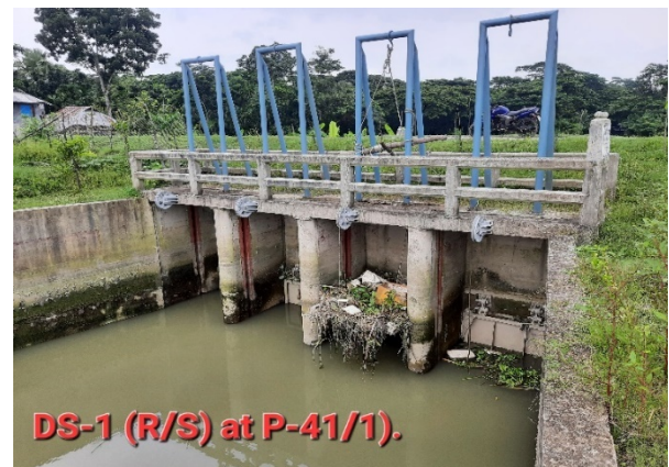
Figure 3-28: Complete Drainage Sluice DS-1 in Polder-41/1
