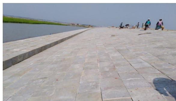
Figure 3-10: Completed Slope Protection Works in Polder-32
