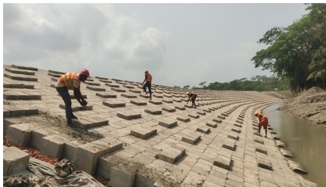
Figure 3-25: Slope protection work for km 32+015-34+300 in Polder-39/2C
