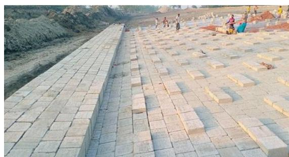
Figure 3-27: Ongoing Slope Protection Works (Polder 40/2), Barguna
