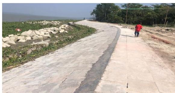
Figure 3-26: Bank Protection with Pitching Works (Polder 39/2C)
