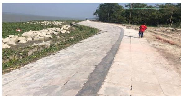
Figure 3-26: Bank Protection with Pitching Works (Polder 39/2C)
