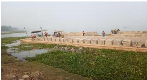
Figure 3-30: Dumping the CC block work at km 53+390 to km 53+418 in Polder 39/2C
