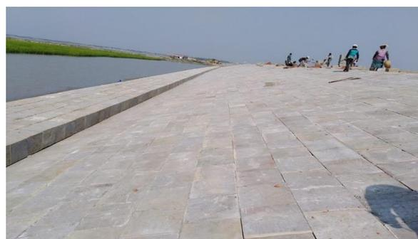
Figure 3-10: Completed Slope Protection Works in Polder-32
