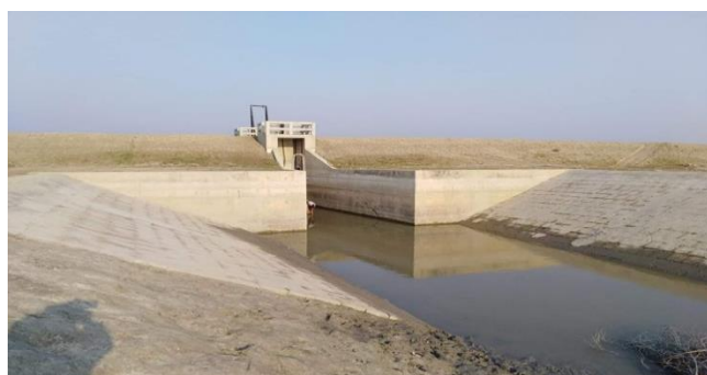
Figure 3-9: Completed DS of Polder-32
