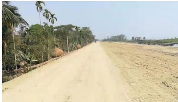
Figure 3-29: Embankment work for K1+750-2+230 in Polder-41/1
