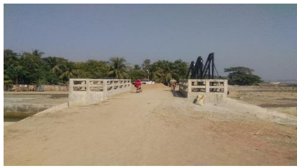
Figure 3-14: Completed DS-10 of Polder-33
