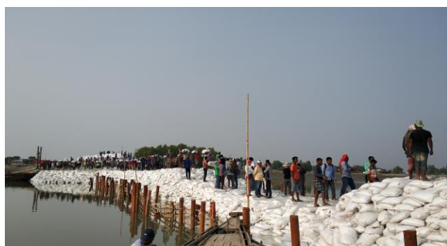
Figure 3-11: Nalian Closure Dam of Polder-32 (completed)
