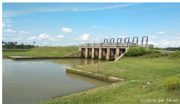
Figure 3-16: DS-6 of Polder-35/3 (Completed)
