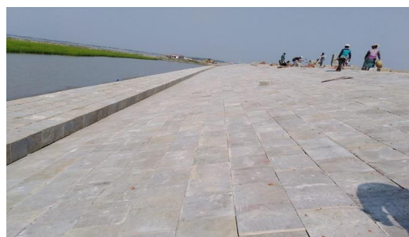
Figure 3-10: Completed Slope Protection Works in Polder-32
