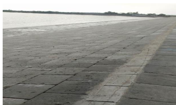
Figure 3-12: Nalian Closure Dam of Polder-32 (completed)
