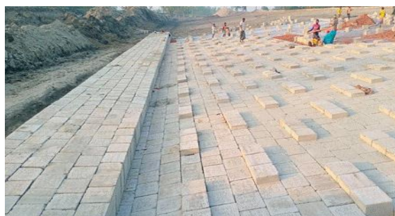
Figure 3-27: Ongoing Slope Protection Works (Polder 40/2), Barguna
