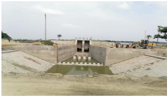
Figure 3-28: Ongoing DS-3 In Polder-43/2C
