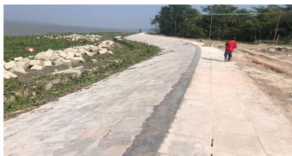
Figure 3-26: Bank Protection with Pitching Works (Polder 39/2C)
