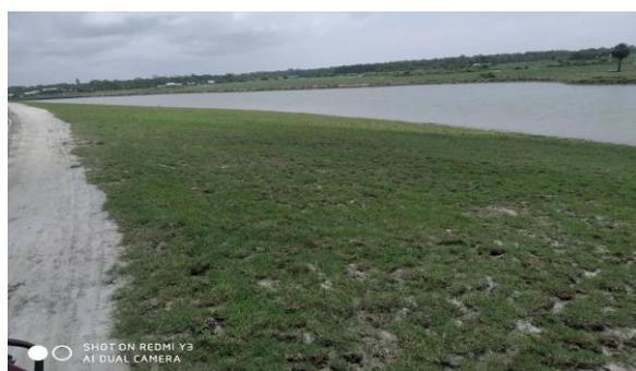
Figure 3-30: Turfing work of Polder-48
