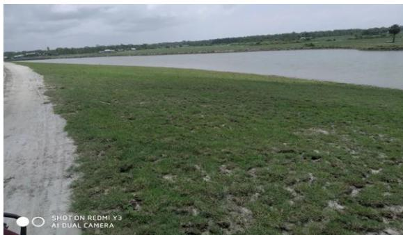
Figure 3-30: Turfing work of Polder-48
