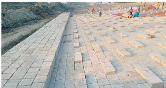
Figure 3-31: Ongoing Slope Protection Works (Polder 40/2), Barguna
