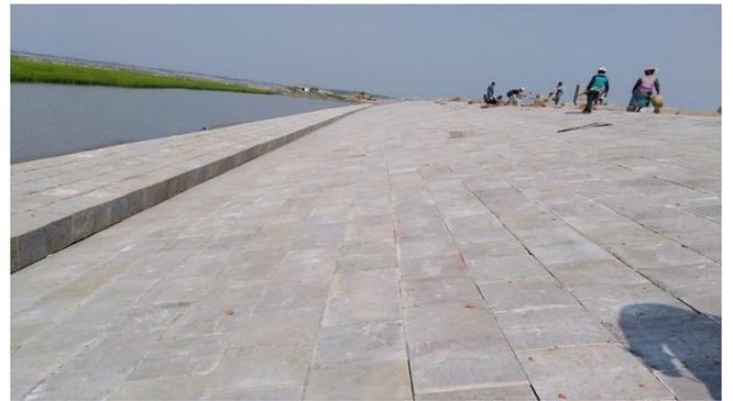
Figure 3-14: Completed Slope Protection Works in Polder-32
