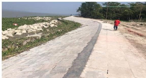
Figure 3-32: Bank Protection with Pitching Works (Polder 39/2C)
