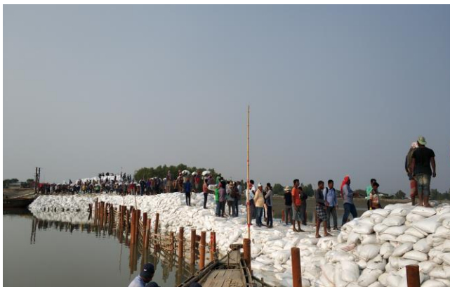
Figure 3-18: Nalian Closure Dam of Polder-32 (ongoing)
