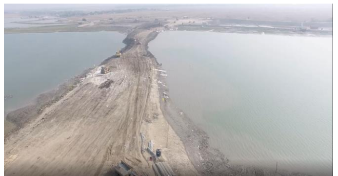
Figure 3-21: Nalian Closure Dam of Polder-32 (ongoing)
