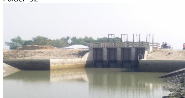
Figure 3-13: Completed Slope Protection Works in Polder-32
