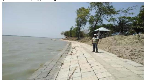
Figure 3-37: Ongoing Bank Protection in Polder-41/1
