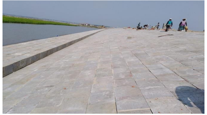
Figure 3-17: Completed Slope Protection Works in Polder-32
