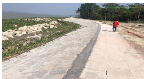
Figure 3-36: Bank Protection with Pitching Works (Polder 39/2C)
