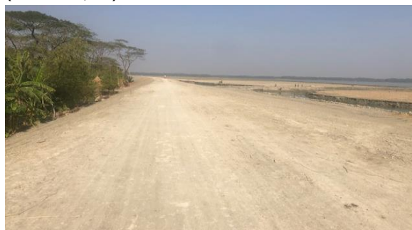
Figure 3-38: Completed Embankment CEIP-1, W/02, Polder 43/2C
