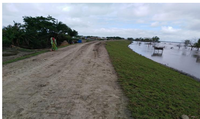
Figure 3-12: Completed Embankment in Polder-32
