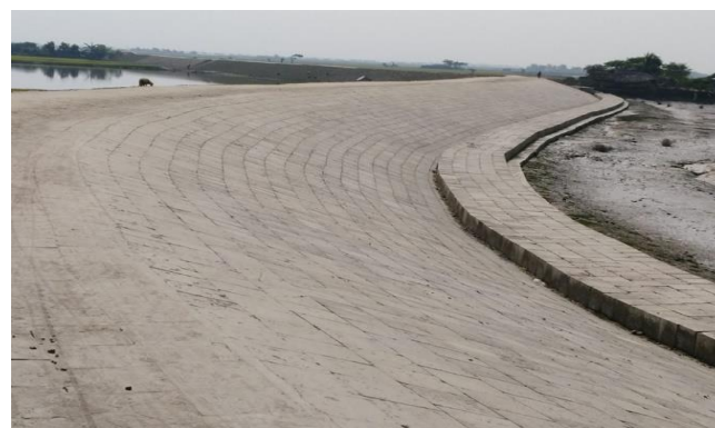
Figure 3-13: Completed Slope Protection Works in Polder-32
