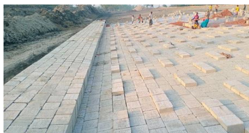
Figure 3-35: Ongoing Slope Protection Works (Polder 40/2), Barguna
