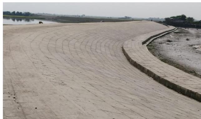
Figure 3-13: Completed Slope Protection Works in Polder-32
