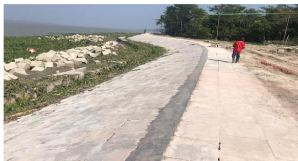
Figure 3-36: Bank Protection with Pitching Works (Polder 39/2C)
