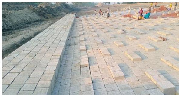
Figure 3-35: Ongoing Slope Protection Works (Polder 40/2), Barguna
