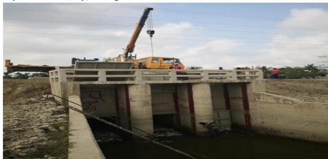
Figure 3-37: Gate installation for DS-1 in Polder 48
