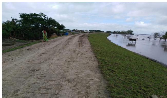
Figure 3-12: Completed Embankment in Polder-32
