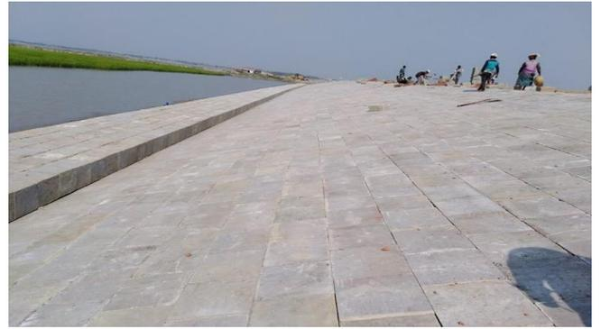
Figure 3-17: Completed Slope Protection Works in Polder-32
