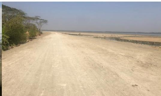
Figure 3-38: Completed Embankment CEIP-1, W/02, Polder 43/2C
