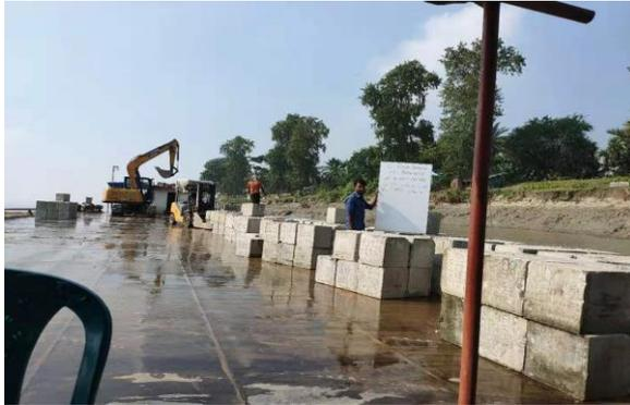
Figure 3-37: Dumping work in Polder-41/1
