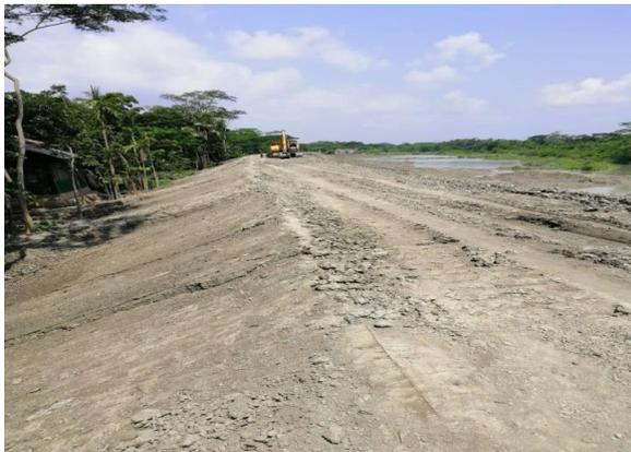
Figure 3-39: Finishing Work for Embankment in Polder 43 /2C
