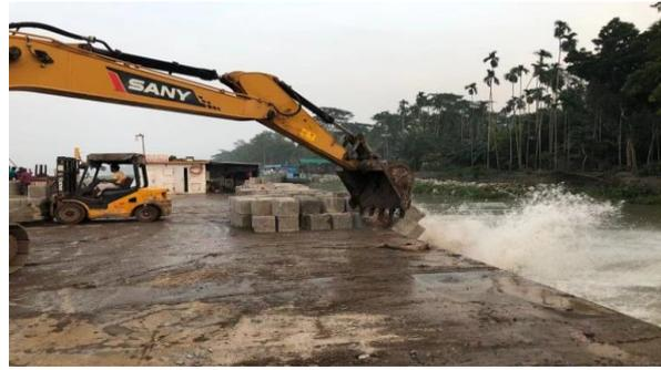
Figure 3-36: Dumping CC Block for river bank protection work (KM51+041-53+418) in Polder 39-2C
