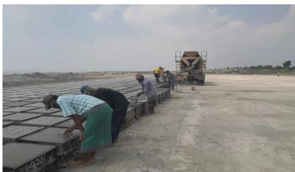
Figure 3-45: CC Block Manufacturing in Polder 48 at yard-3
