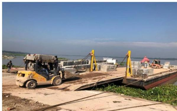
Figure 3-44: Loading CC Block on the berge in Polder-39/2C
