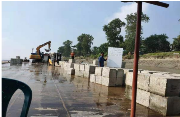
Figure 3-59: Dumping work in Polder-41/1
