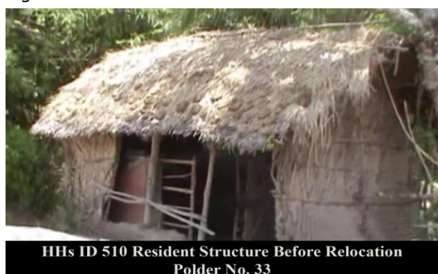
Figure 3-3: HH 510 Before relocation of Polder-33
