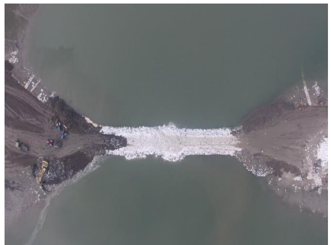
Figure 3-41: Nalian Closure Dam of Polder-32
