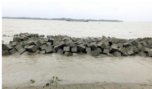
Figure 3-57: Dumping the CC Block at Km 51 in Polder 39-2C
