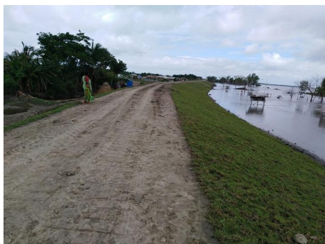
Figure 3-34: Completed Embankment in Polder-32
