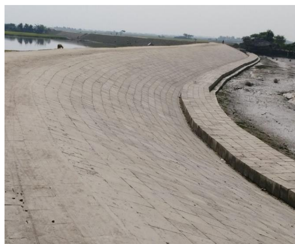
Figure 3-35: Completed Slope Protection Works in Polder-32
