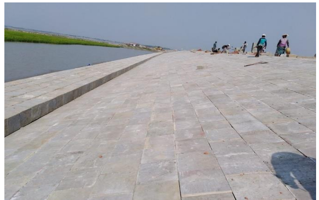
Figure 3-39: Completed Slope Protection Works in Polder-32
