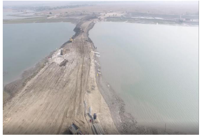
Figure 3-43: Nalian Closure Dam of Polder-32
