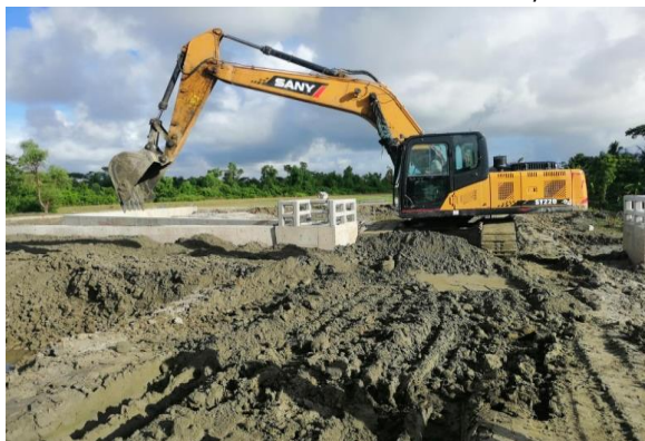
Figure 3-63: Back fill & Repair of access road for DS-01 in Polder 47/2
