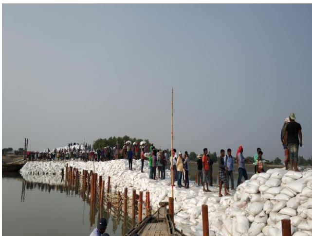
Figure 3-40: Nalian Closure Dam of Polder-32
