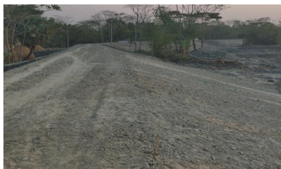
Figure 3-68: Embankment work for Km 0-0+500 in Polder 43-2C
