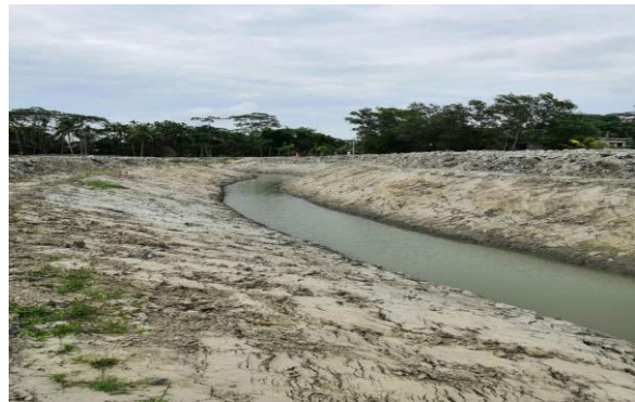
Figure 3-60: Completed Section Drainage Channel for DS-07 in Polder 43/2C
