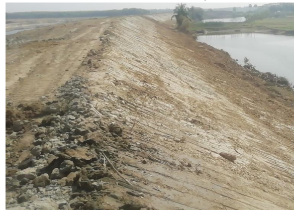
Figure 3-62: Embankment work for K17 in Polder 48
