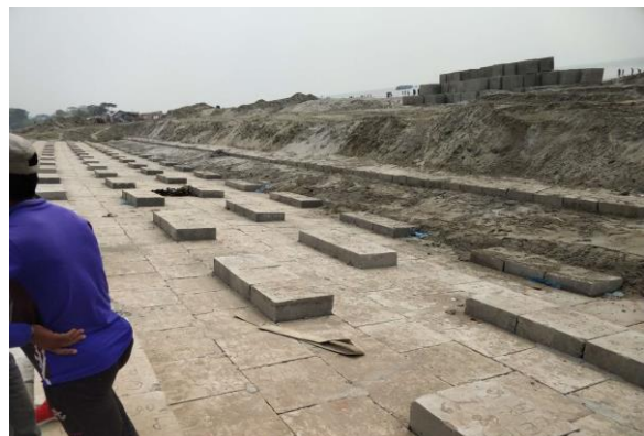
Figure 3-64: Slope Protection work for K30 in Polder 48
