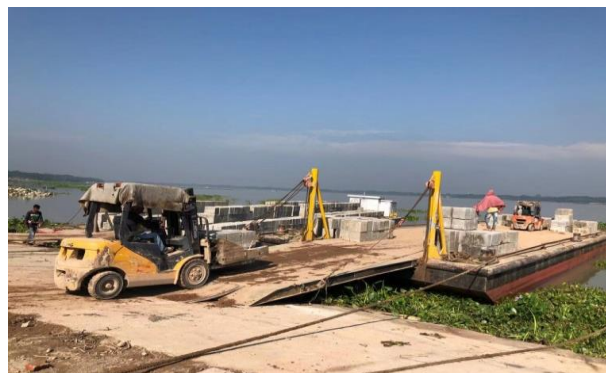
Figure 3-66: Loading CC Block on the berge in Polder 39-2C
