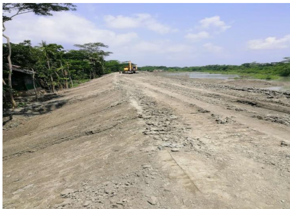
Figure 3-61: Earth Work for Embankment KM1+000 to Km2+000 in Polder 43 /2C
