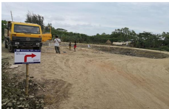
Figure 3-65: Install of Waring Tape for FS-3 in Polder 48
