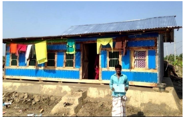
HHs ID 771 Resident Structure After Relocation
