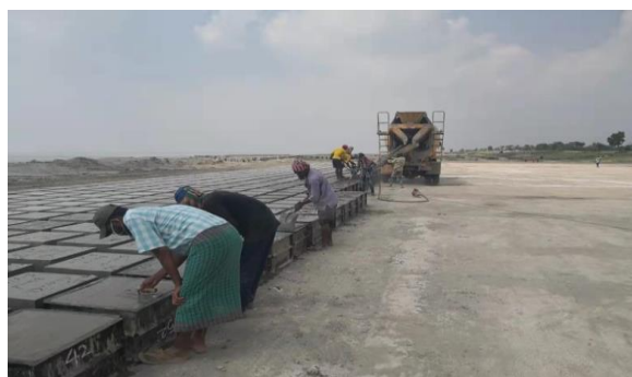
Figure 3-67: CC Block Manufacturing in Polder 48 at yard-3
